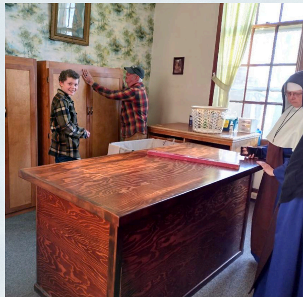
Mr. Murry's apprentice, William, helped to build these cabinets. Since they were for the Sisters' cloister, he gets a sneak peek of the convent during installation.
